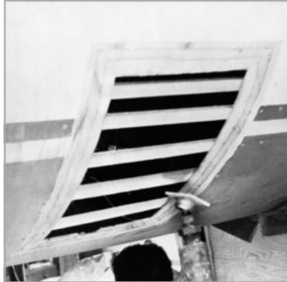
Figure 5-16 Bevel the edges and fasten temporary stringers to the back of the opening.
